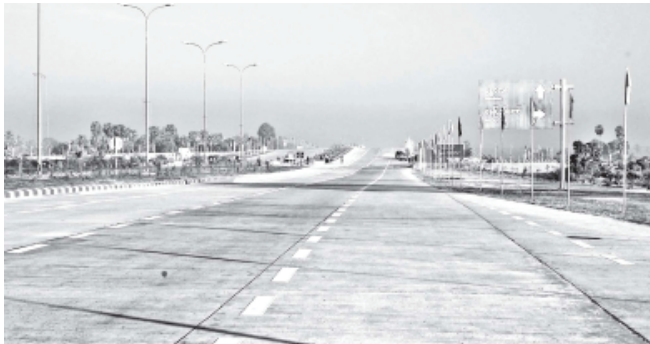
A section of Yangon-Mandalay Highway (Nay Pyi Taw-Mandalay section) constructed in line with ASEAN norms and international designs.
