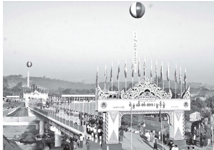
Yenwe Chaung Bridge over Yenwe Creek in Kyaukdaga Township of Bago District was opened on 28 January to help access between the eastern and western parts of Bago Region. (News reported)
