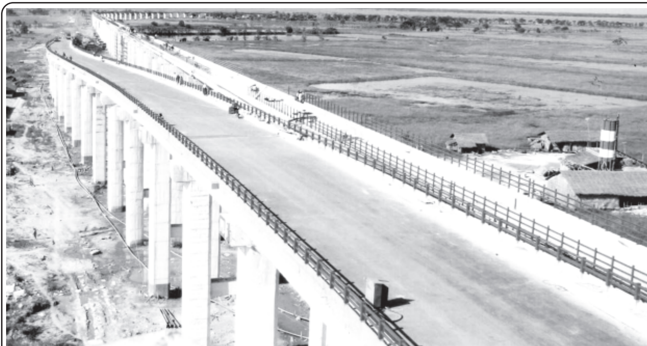
Approach road and approach bridge of Ayeyawady Bridge (Nyaungdon) seen on 29 th October, 2011.
