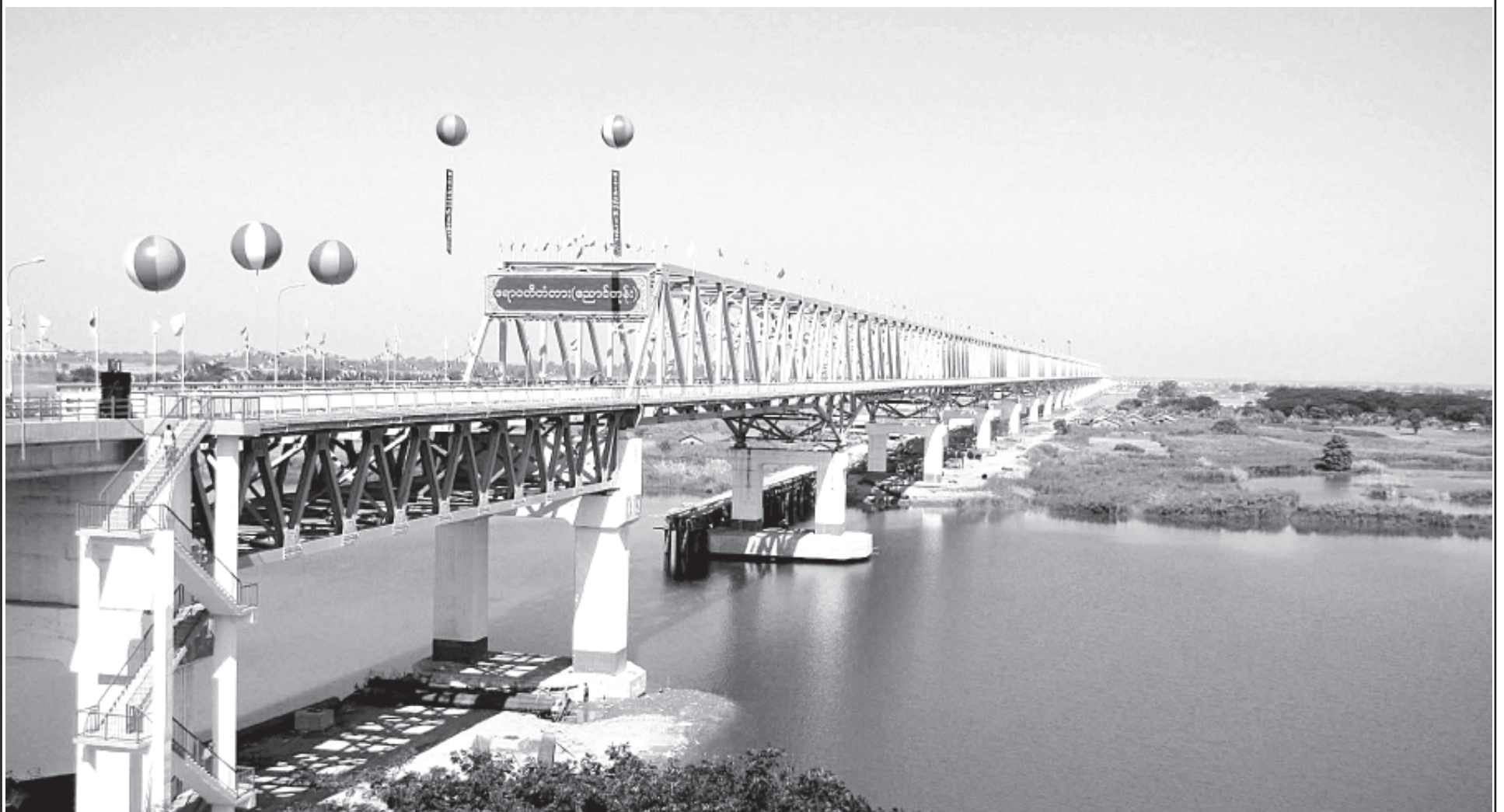
Ayeyawady Bridge (Nyaungdon), the eighth bridge opened in the time of new government of the Republic of the Union of Myanmar.
