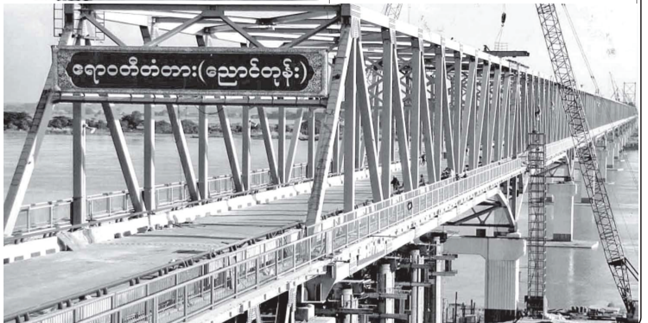
Construction site of Ayeyawady Bridge (Nyaungdon) on 12 th August, 2011.
