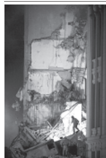
A firefighter searches for survivors in a building that collapsed in downtown Rio de Janeiro, Brazil, on 25 Jan, 2012.—INTERNET
