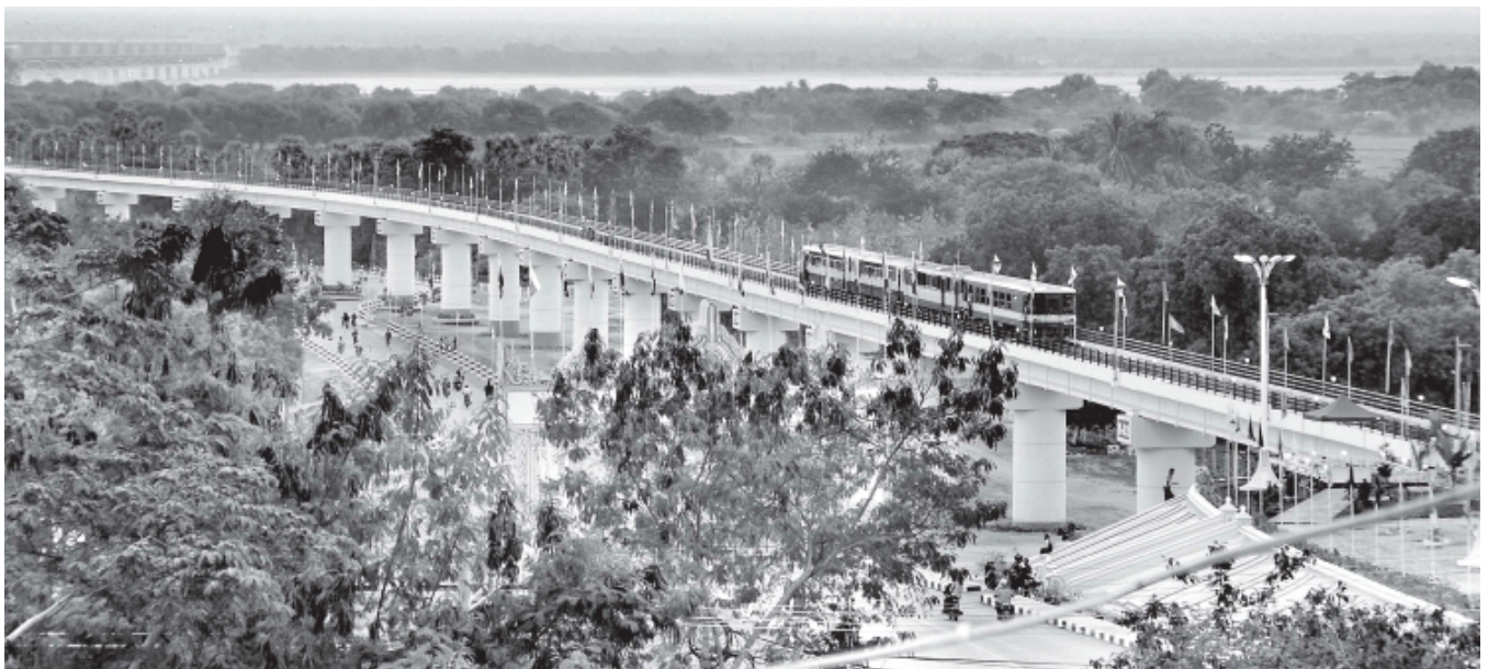
Photo shows Ayeyawady Bridge (Pakokku) which was opened on 31-12-2011 is the longest facility of its kind in Myanmar.—MNA
