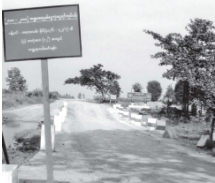
Overpass constructed by Road Special Group No. 11 at Kalay-Gangaw border.
