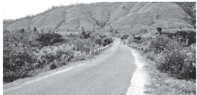
Gangaw-Kalay Road constructed by Road Special Group No. 11
