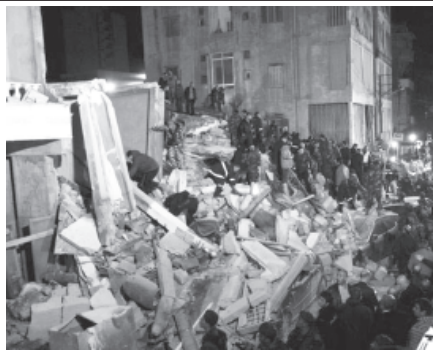
Lebanese people and Red Cross members search through the rubble of a six-storey building that collapsed in Beirut's Ashrafieh neighbourhood.
