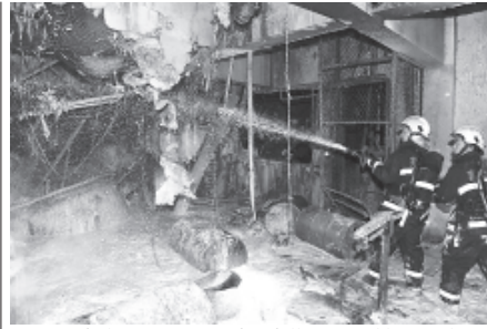
Fire fighters put out a fire following a blast at the Xiangyang chemical plant in the Nanhua District of Jiaying, east China's Zhejiang Province, on 4 Jan, 2011. The blast occurred Wednesday night, leaving three workers dead and four others injured, the Nanhua District Information Office said on 5 Jan.—XINHUA
