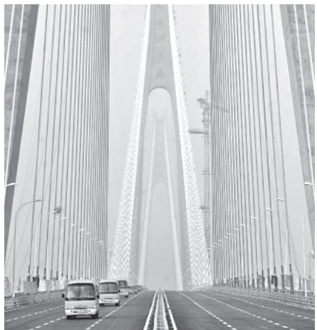
Photo taken on 31 Dec, 2011 shows the Erqi Yangtze River Bridge in Wuhan, the capital of central China’s Hubei Province. The Erqi Yangtze River Bridge, the seventh Yangtze River Bridge, was completed and opened to traffic on Saturday. The bridge, 6,507 meters in total length with two main 616-meter spans, was both the three-bridgehead cable-stayed and composite-beam cable-stayed bridge with the world’s largest span.—XINHUA
