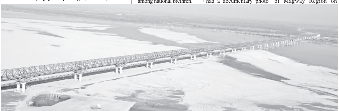
Aerial view of Ayeyawady Bridge (Pakokku).—MNA
