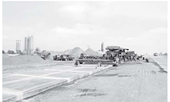
Paving concrete on Nay Pyi Taw-Mandalay road section in progress.
