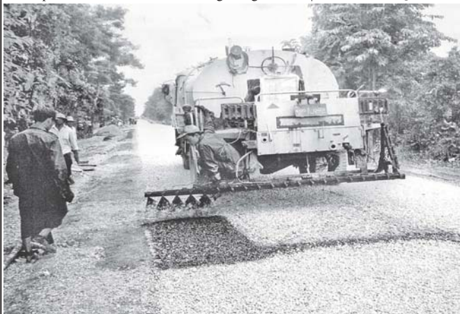
A Tar Spraying Vehicle seen at construction work at mile post No. 166/3 on Pathein-Monywa Road.
