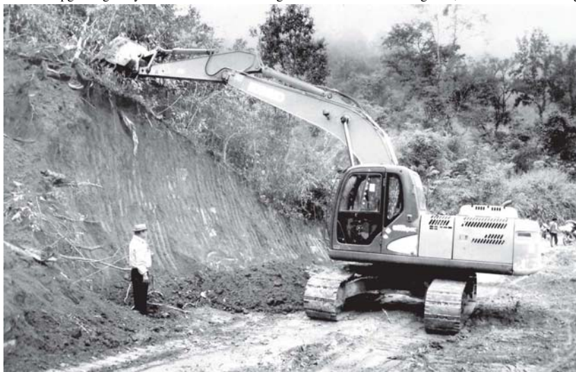
Heavy machinery expanding Kutkai-Tamoenye-Monesi-Tarpa 18 th -mile junction (Tarshwehtan) Road to be a 34 feet wide facility.
