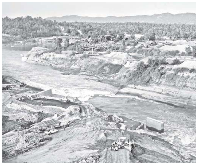
Temporary water course of Mone Creek seen in construction site of Kyeeohn-kyeewa Multi-purpose Dam.
