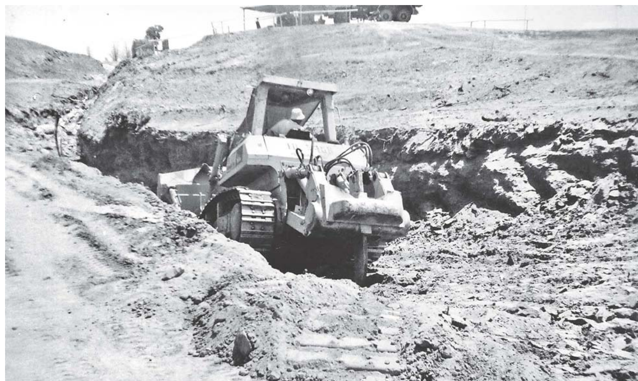
A bulldozer at work in building of spillway of Motkhar Dam Project.
