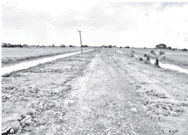
Groundwork is being carried out to upgrade Pathein-Ngapudaw Road to a 34 feet wide tarred facility.
