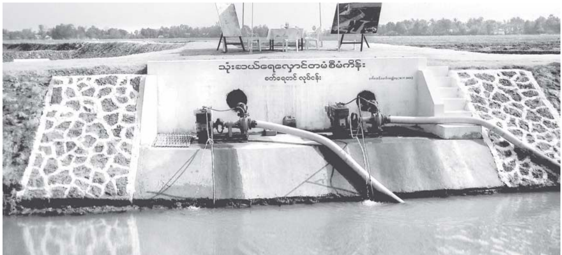
Two motor pumps to supply irrigation water to 200 acres of farmlands.
