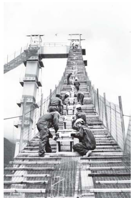
Myanmar engineers of Public Works installing main cable at Leinli Suspension Bridge.
