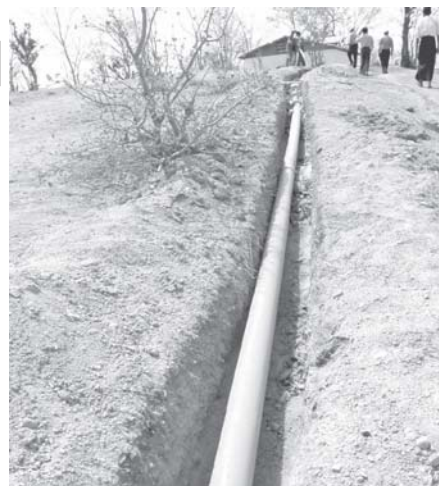
Water pipelines being laid onto Thein Hill.
