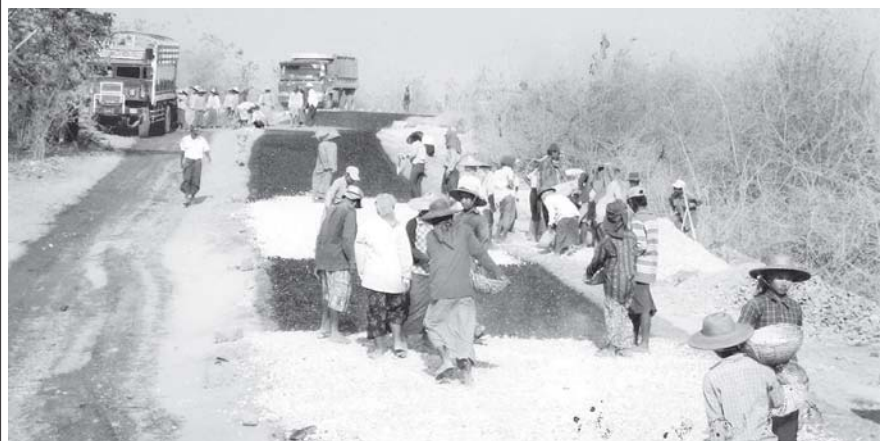
Workers at the tarmacking sections on Patheingyi-Thalakhwa-Mawtinsoon Road. (See page 7)
