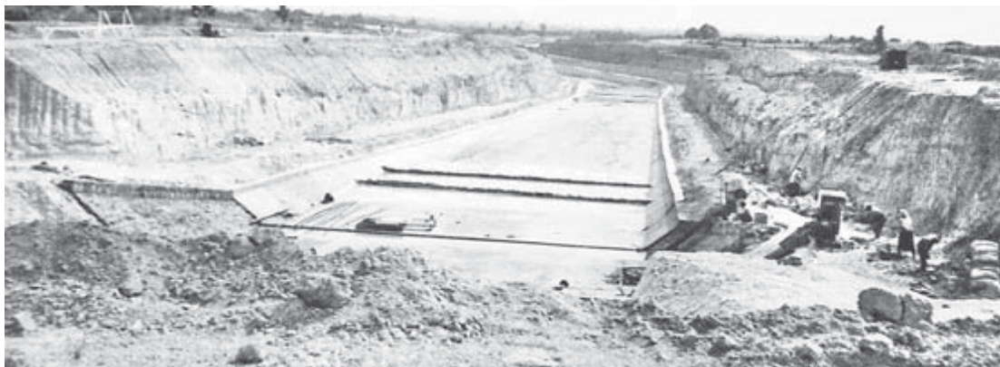
Photo shows spillway of Theinyin Dam under construction in Kanbalu Township of Sagaing Division.
