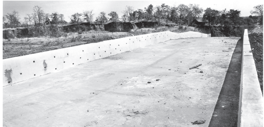
Photo shows 40 feet wide concrete main spillway of Wunyu Dam.
