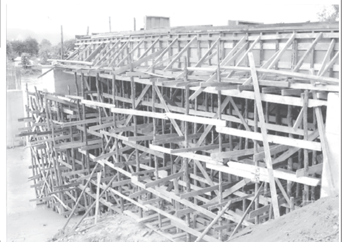
The approach structure and pillars under construction at Hsipaw Bridge Project.
