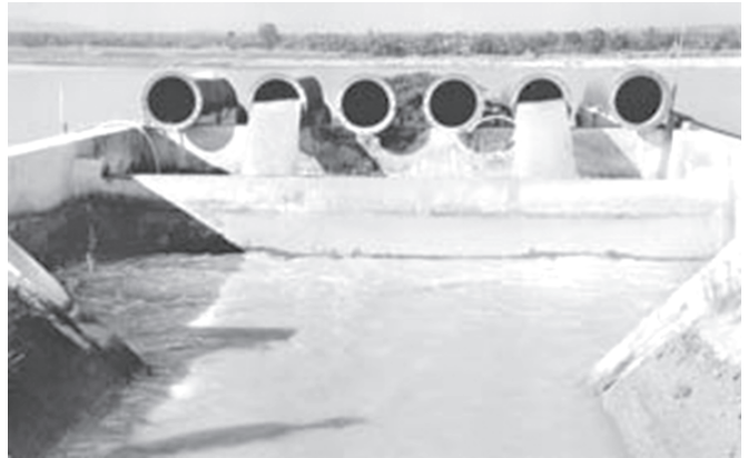
Pipes to pump water from Chindwin River to main canal.
