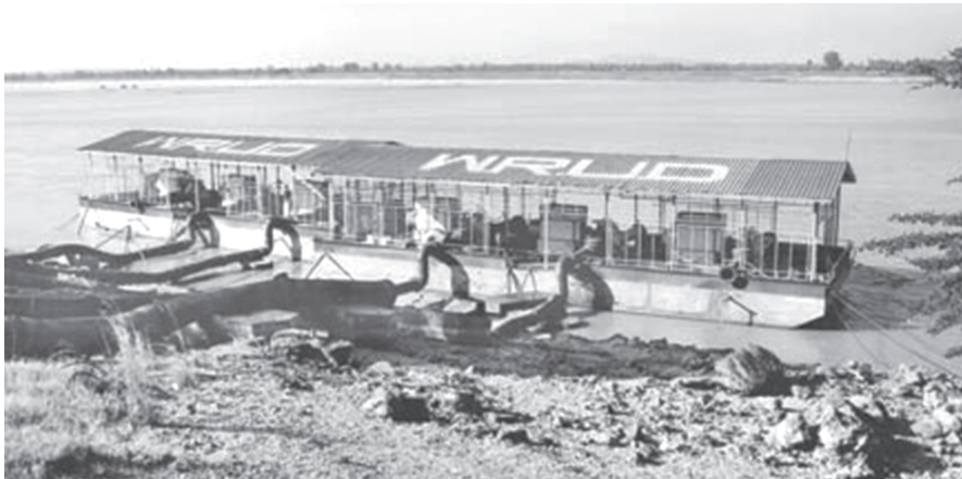
Pipes to pump water from Chindwin River to main canal.
