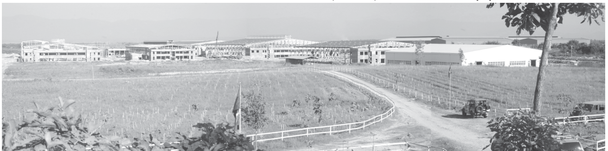
Construction tasks of Thagara Industrial Region Project in progress.—MNA
