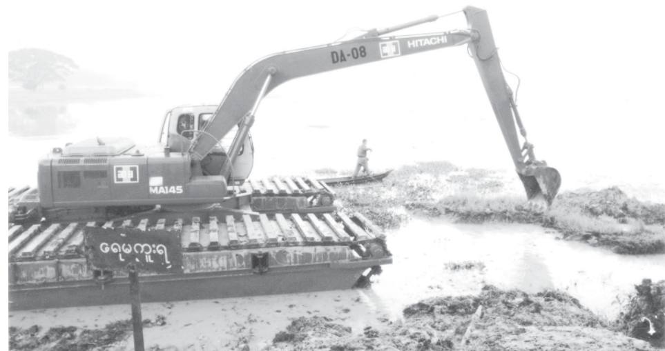
A machinery dredging Inya Lake to make the lake deeper and water cleaner. — YCDC
