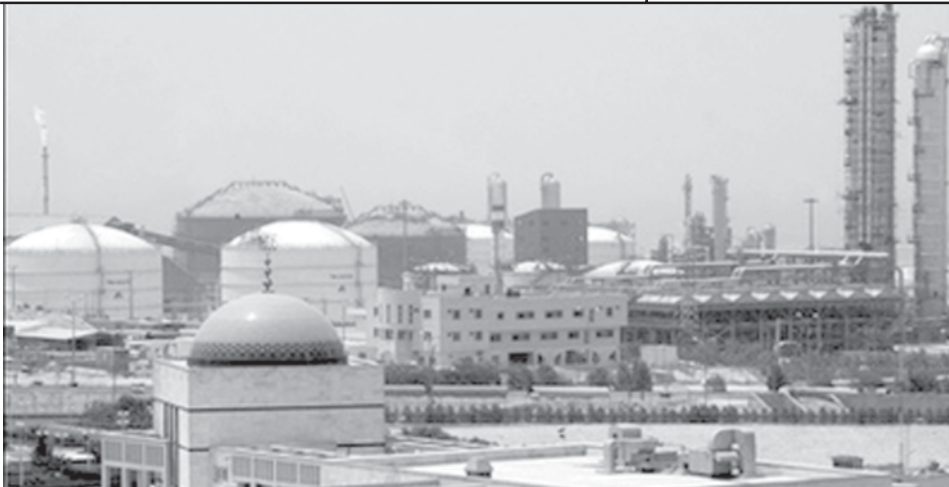
The south Pars gas field in Asaluyeh, July 2007. Iran and Malaysia on Wednesday signed a multi-billion dollar contract to develop two offshore Iranian gas fields.—INTERNET
