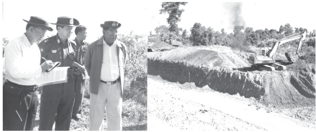
Minister Maj-Gen Aung Min inspects earth works of Katha-Bhamo railroad section. RAILWAY
