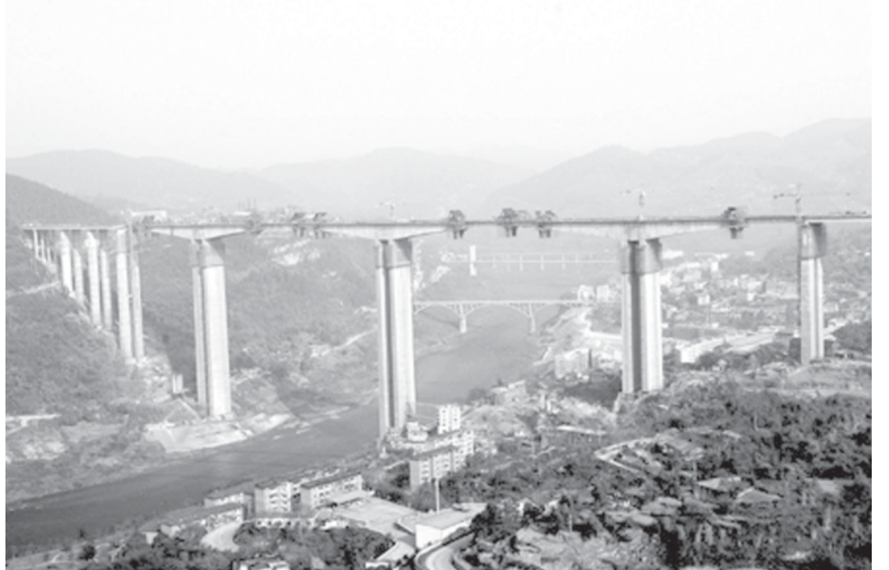
The Wujiang Mega Bridge is seen under construction over the Wujiang River near Guiyang, Southwest China's Guizhou Province, on 11 Dec, 2007. The tallest pier of the 1,452-metre-long bridge stands 173.5 metres high, and the bridge will open to traffic before the new year. —XINHUA
