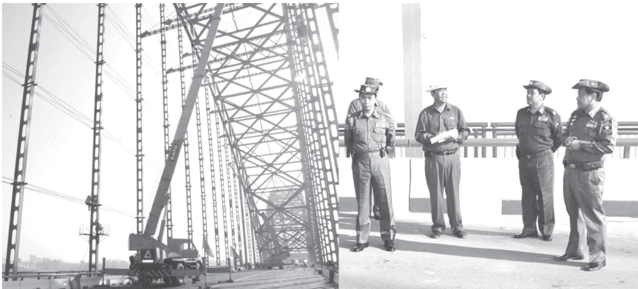
□Lt-Gen Ye Myint of Ministry of Defence inspects construction tasks of Ayeyawady Bridge (Yadanabon).— MNA
