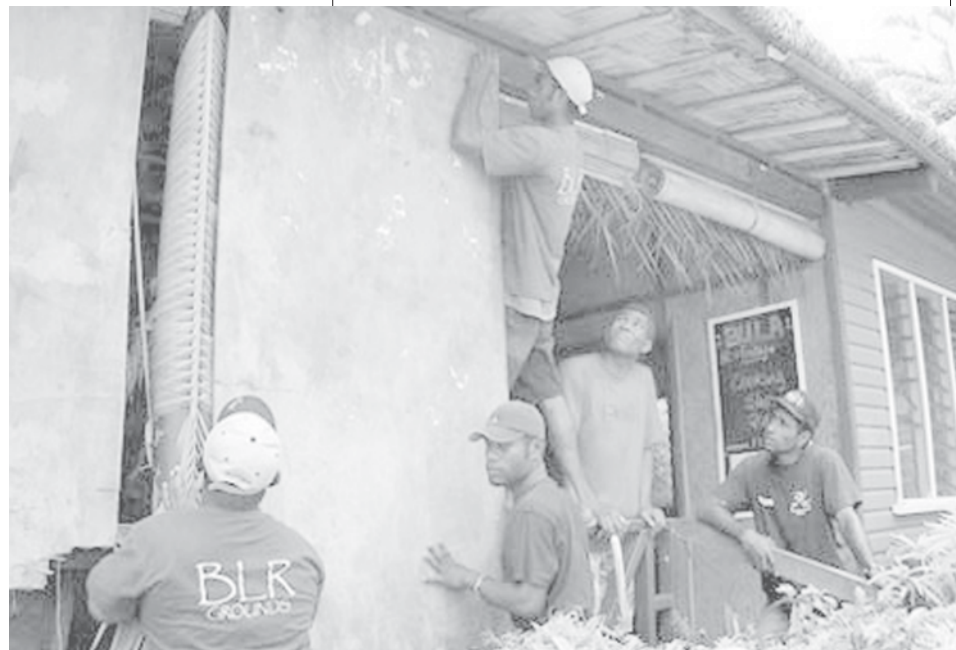
Workers at the Bega Lagoon Resort in Fiji Islands putting up sheets of plywood as they prepare for Tropical Cyclone Daman. —INTERNET
