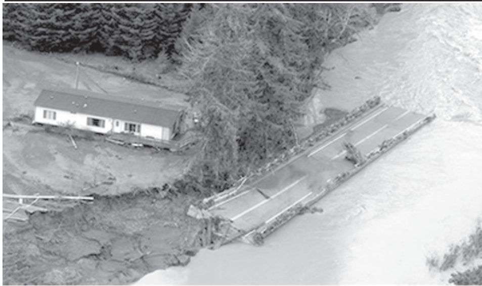
A piece of broken roadway lies in a muddy river in rural Lewis County, on 6 Dec, 2007. Floodwaters were receding across southwestern Washington state on Thursday, rescue and evacuation work ended and lights were coming back on in thousands of homes and businesses. —INTERNET
