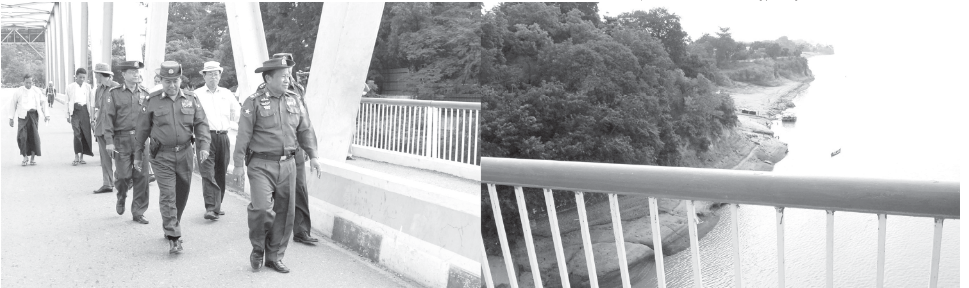
Lt-Gen Ye Myint of the Ministry of Defence looks into maintenance of Ayeyawady Bridge (Anawrahta) in Chauk. —MNA
