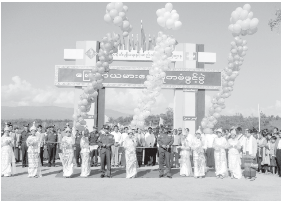
Commander Brig-Gen Myint Soe and Minister Maj-Gen Htay Oo formally open North Yama Supporting Dam in Pale Township.—MNA
