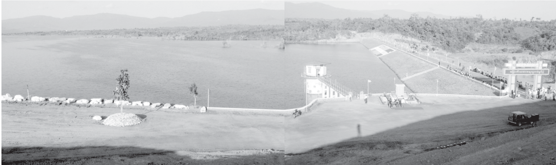
North Yama Supporting Dam in Pale Township seen after opening ceremony of the dam.—MNA
