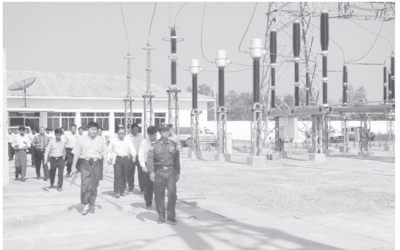
Minister Maj-Gen Khin Maung Myint at Myaungdagar Main Power Station in Hmawby.
