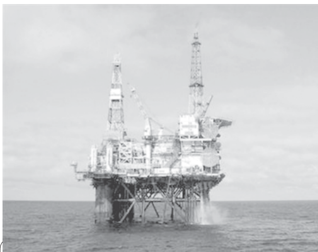
The North Sea oil platform Thistle Alpha is seen in this undated handout photograph, received in London on 25 Nov, 2007. The platform was briefly evacuated on 25 Nov after a fire broke out on board, rescue officials said.
