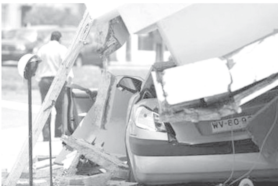
A crushed car is seen under a roof that collapsed during earthquake in Antofagasta, 1,360km northwest of Santiago on 14 Nov, 2007. A powerful earthquake hit mineral-rich northern Chile on Wednesday, killing at least two people, injuring more than 100 and halting output at some of the world's largest copper mines. —INTERNET
