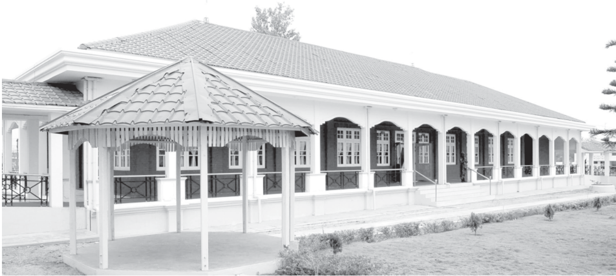
The (300)-bed hospital in PyinOoLwin.
