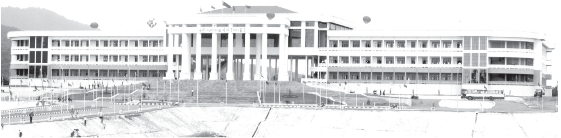
The three-storey main building of Lashio Technological University.
