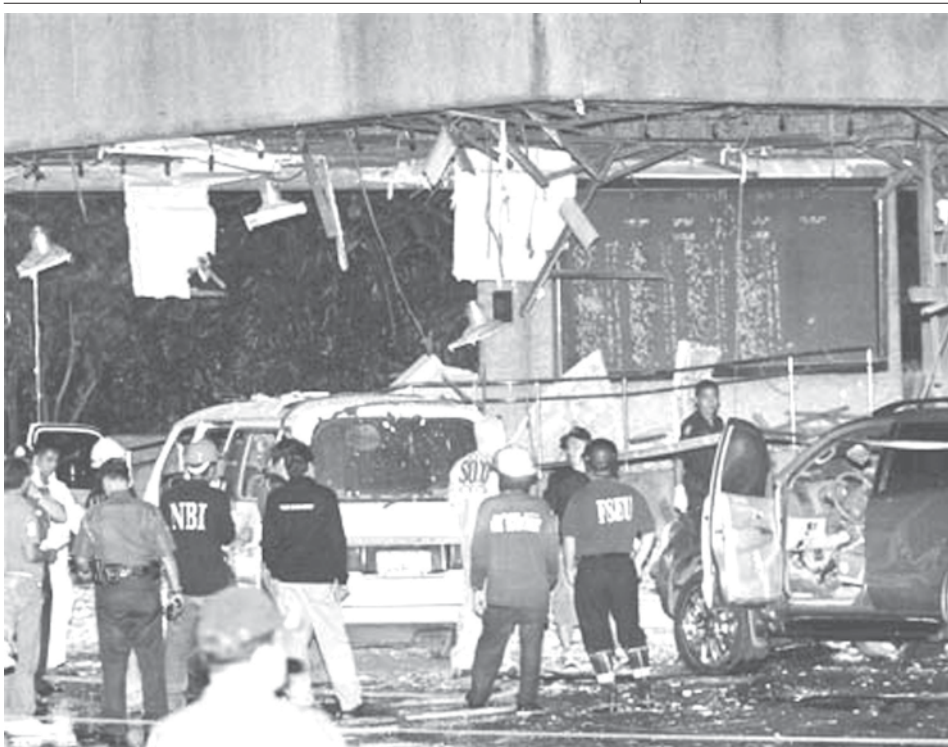
Police investigators inspect the explosion site at the entrance of the Congress building in Manila, on 13 Nov, 2007. The bomb rips through a section of the Philippine House of representatives, killing two persons and injuring at least ten others. —INTERNET
