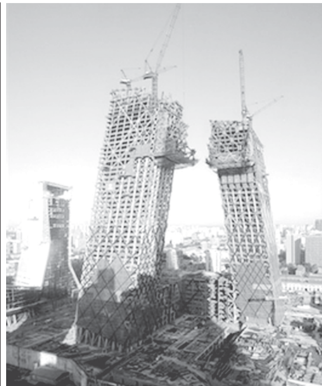
The leaning towers of the new China Central Television headquarters building are seen nearing their full height in Beijing Wednesday Oct. 31, 2007. The two towers are expected to be connected within the coming months. The building will consist of two angled towers connected at the top to form a continuous loop of horizontal and vertical sections, when completed in 2008, in time for the Beijing Olympic Games. The spectacular 230 meter (755 foot) building, one of Beijing’s tallest, will house more than 10,000 staff.—INTERNET
