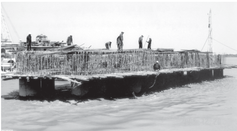
Workers at work to cap Pillar No 13.
