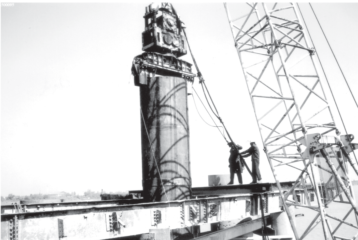
Two workers driving a stand pipe.
