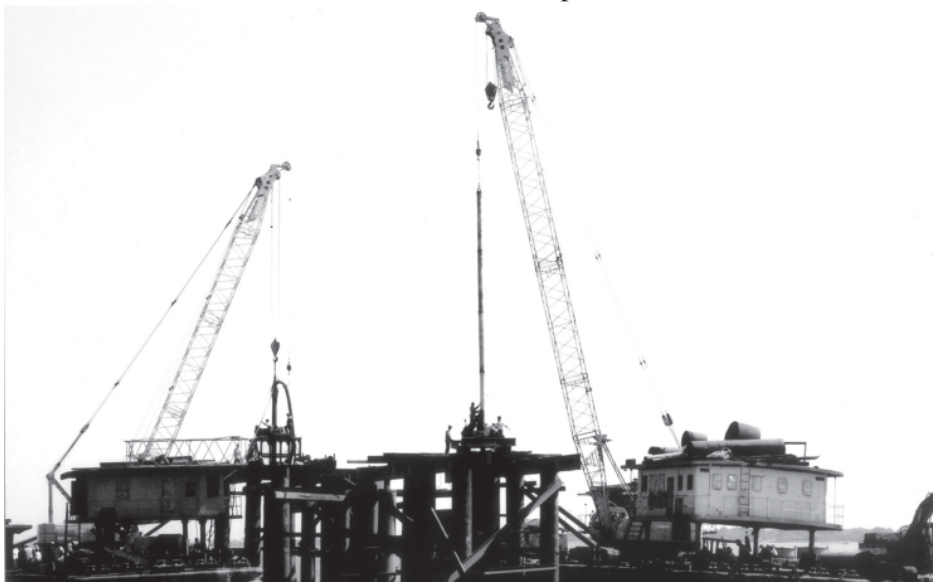
Two RCD machines are used in tandem to drill two holes for setting piles at main pillar No 12.
