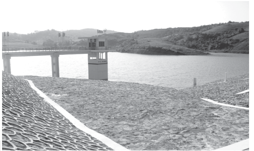
Newly-opened Sitha Supporting Dam in PyinOoLwin.—MNA
