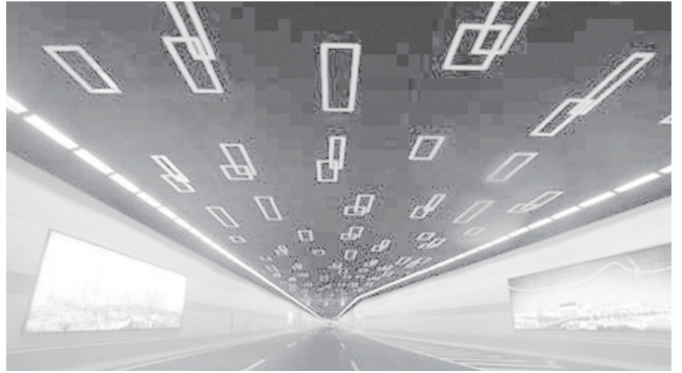
A handout photo shows the Dushuhu Tunnel of Suzhou, east China's Jiangsu Province. The construction of Dushuhu Tunnel, measuring 7.37-kilometre-long, has come to the end, which will open soon. — INTERNET
