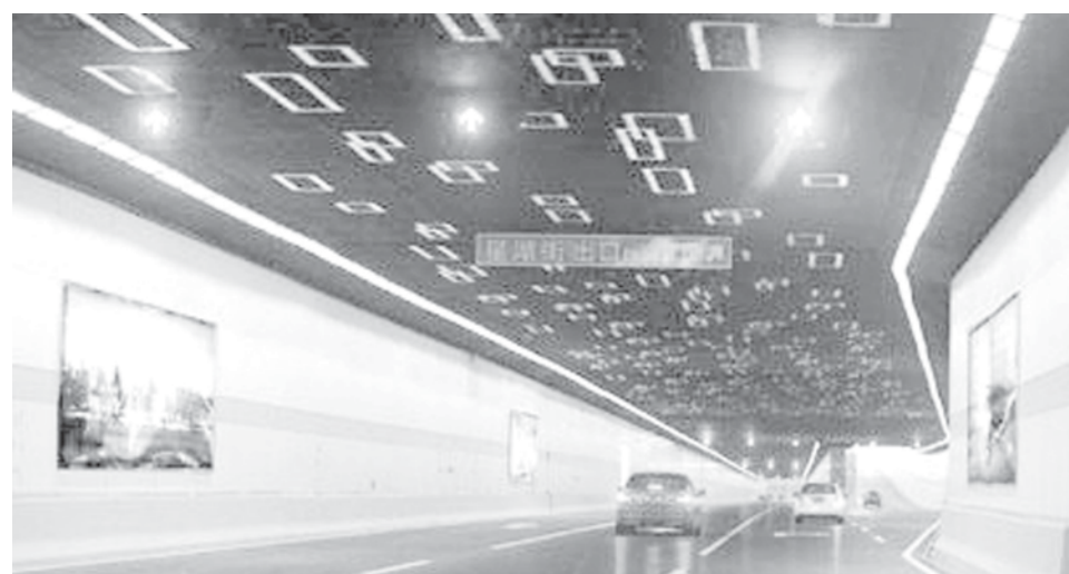
Vehicles move along a 3.46 km-long tunnel under the Dushuhu Lake in Suzhou, East Chin's Jiangsu Province on 10 Oct, 2007. The tunnel is part of the 7.37 km-long Dushuhu bridge and tunnel project, which opened to traffic on Wednesday after more than one year of construction. The tunnel is longest of its kind in China.—INTERNET
