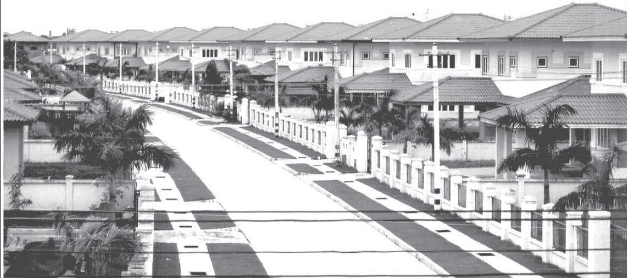
Single-unit houses in Hlinethaya Township.
