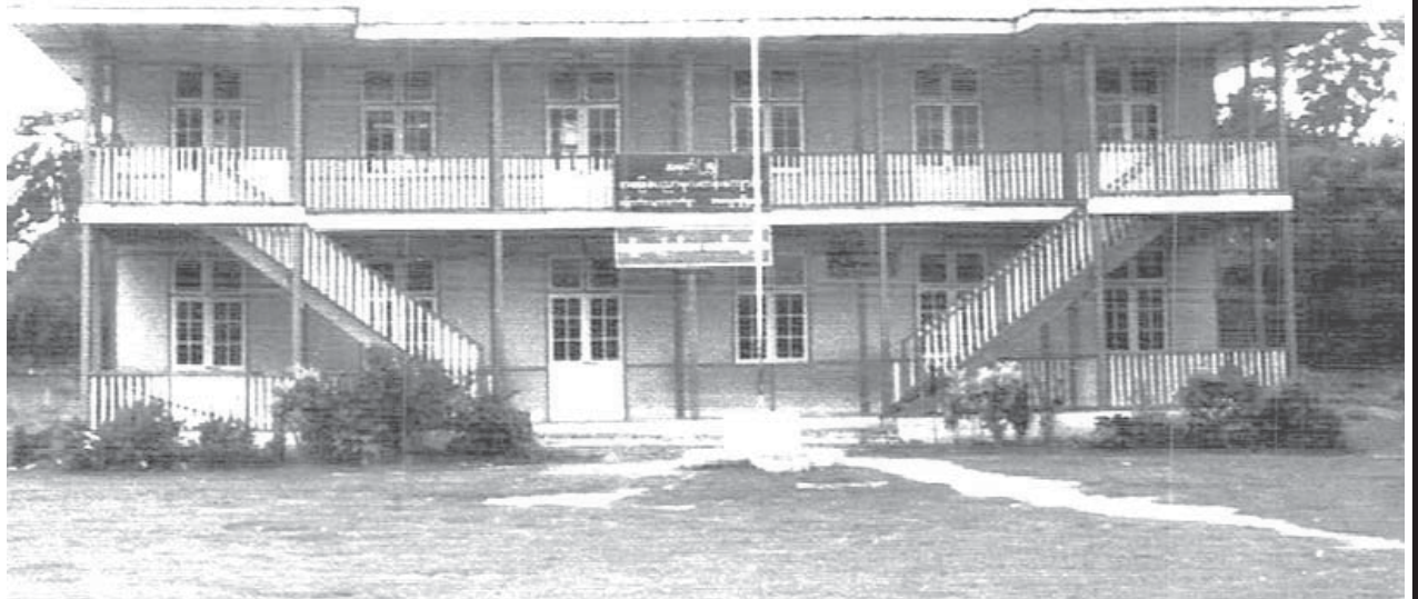
A primary school in Chaukthwaythauk Village in Amarapura Township.
