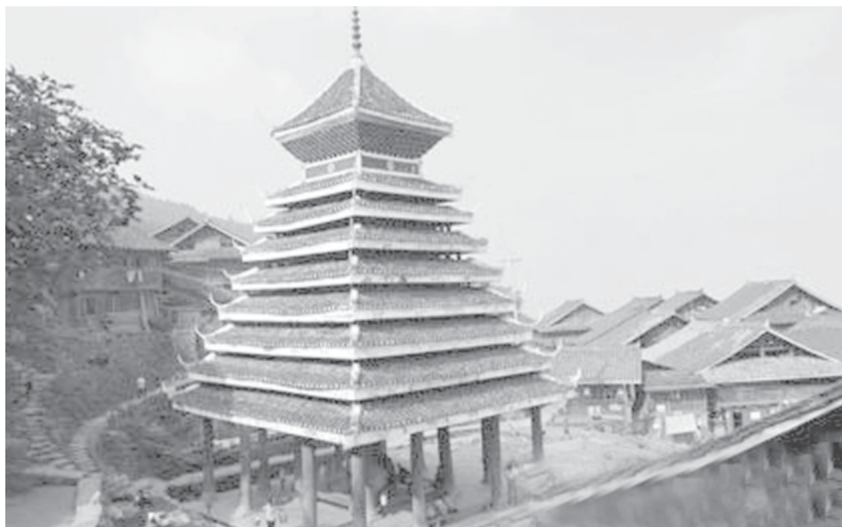
Photo taken on 7 Oct, 2007 shows the Tangan Gulou, or drum tower, in Zhaoxing, Liping county of southwest China's Guizhou Province. Gulou, special towers made of wood without the aid of nails, are symbols of
