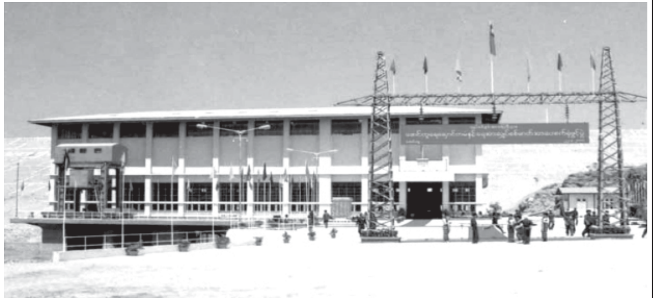
Zaungtu Hydroelectric power station in Bago Division.
