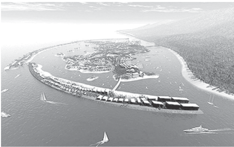
This computer generated hand out image shows a plan of a luxury island which will built in the Black Sea, outside the Russian resort of Sochi. Russian developers outlined plans on 21 Sept, 2007 for a 350-hectare artificial island in the shape of Russia to be built off the Black Sea coast near the future Olympic venue Sochi.—INTERNET
