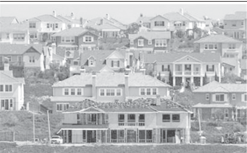
Construction work continues on new homes in Carlsbad, California on 18 Sept, 2007. While California suffers in the housing crisis, the economy of nearby Washington state is flourishing with strong job growth and some of the highest appreciation in home prices in the nation. — INTERNET
