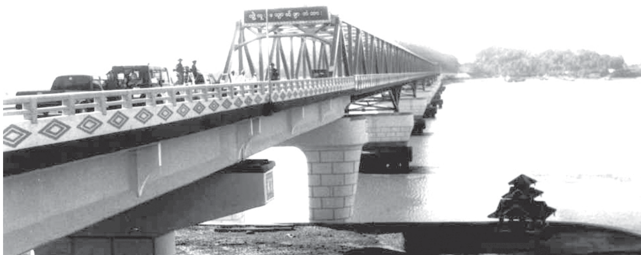
Kyweku-Kyaukphya Bridge constructed by Public Works of the Ministry of Construction in Myeik, Taninthayi Division.
