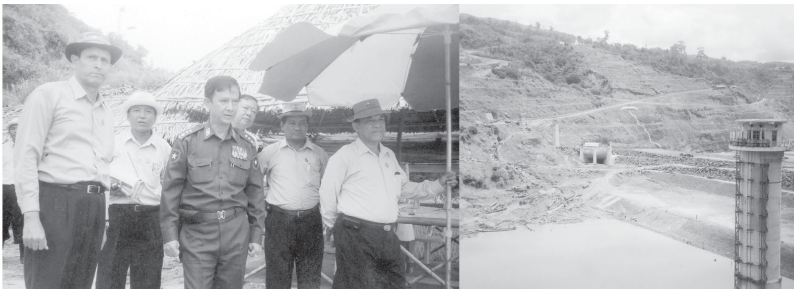
Minister Col Zaw Min inspects construction tasks of Kunchaung Hydropower Project.— E P - 1
