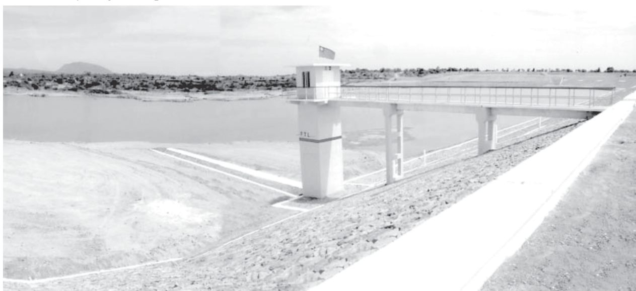
Gwegyo Dam, 15,000 feet long and 57 feet high is built on Hsinmawin Creek in Yesagyo Township, Magway Division.
