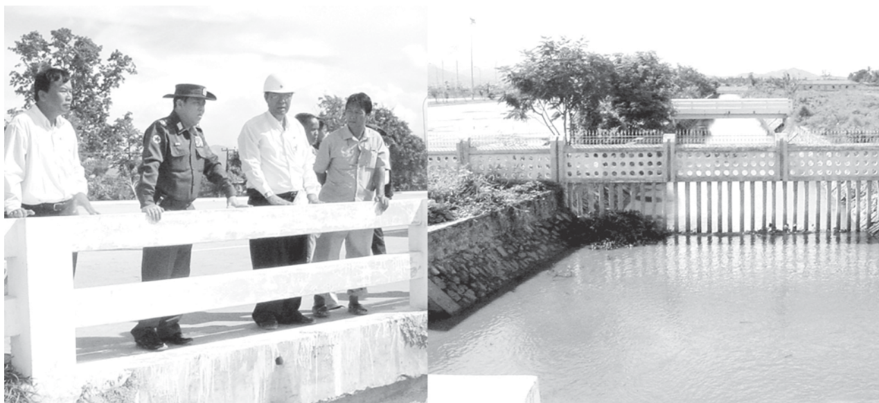
Commander Maj-Gen Wai Lwin inspects sluice gate of Yezin Dam.—MNA
