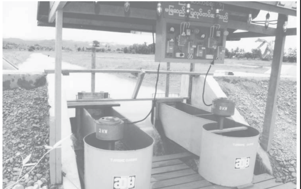
2KW-AMP machines are generating power to light the whole Mhyin-wataung village lying near Mya Mya Dam.
